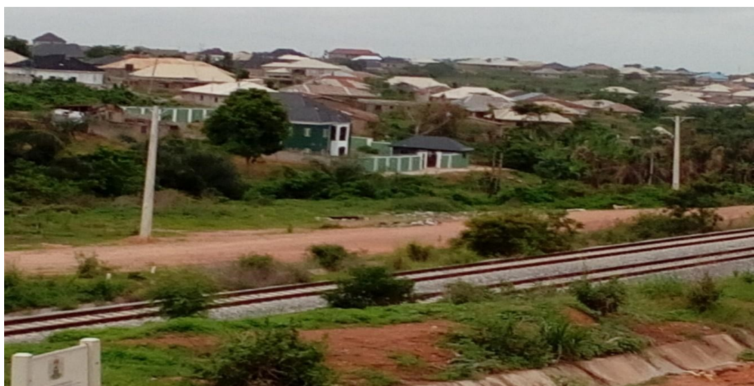
Figure 4.4. Railway Infrastructure and Rapid Development in Idi Igbaro Ologuneru Area Source: Fieldwork 2023
